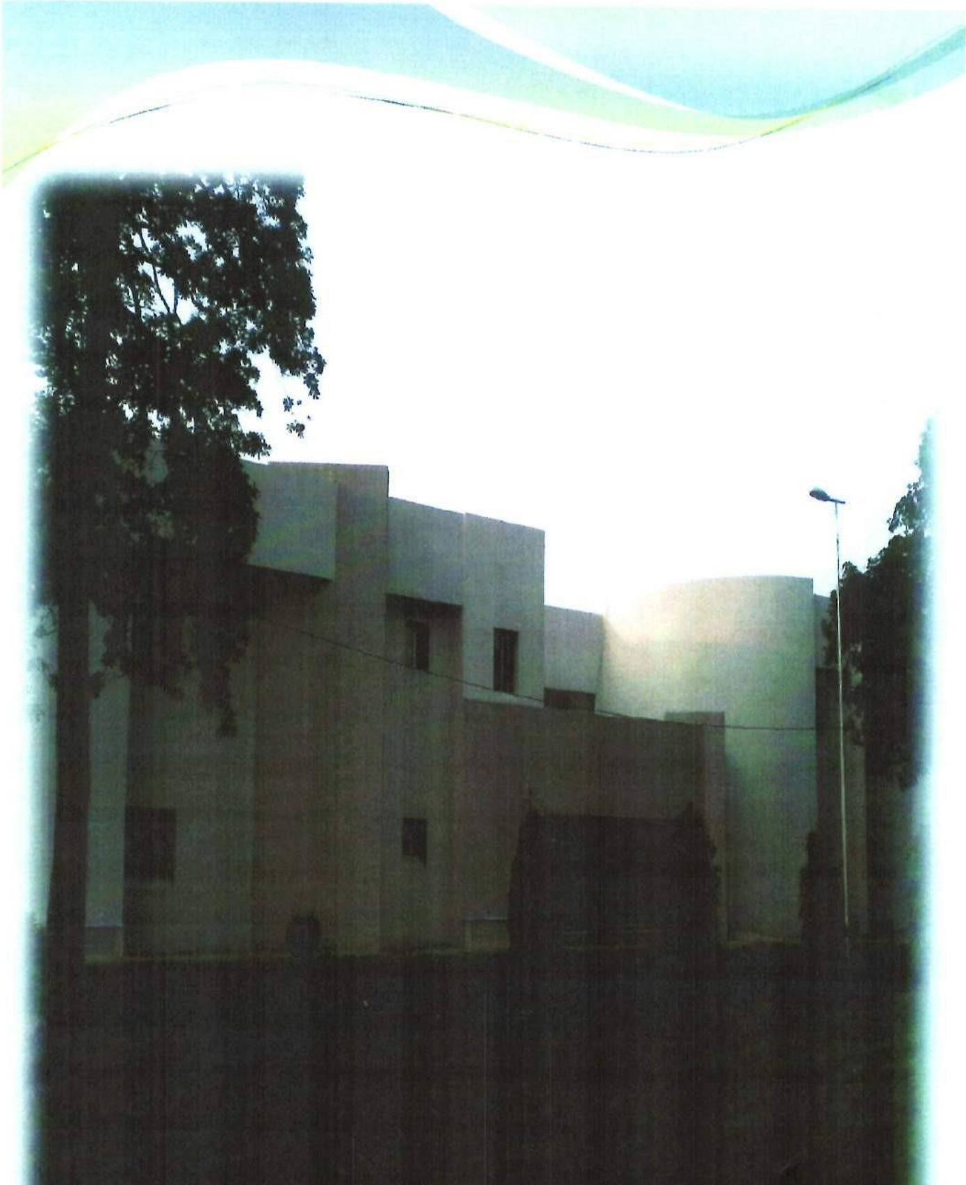
OPD COMPLEX CMH JHELUM
